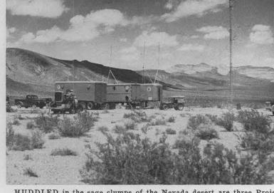
HUDDLED in the sage clumps of the Nevada desert are three Project Outcast trailers. Shown here are two telemetering labs and a mobile photo processing laboratory for on-the-spot development of field test results and photographic material.
